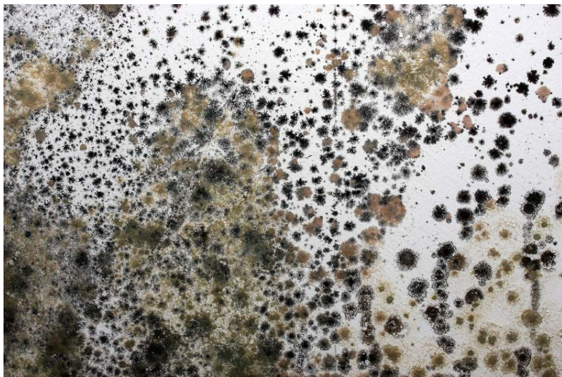
Varied colours of mould colonies on the same material, drywall
